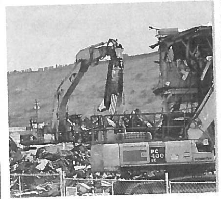
DEMOLISHING SUPPORT FACILITIES
