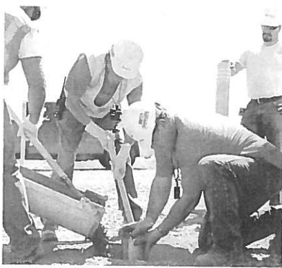
CREATING A WELL TO EXTRACT CONTAMINATED WATER
